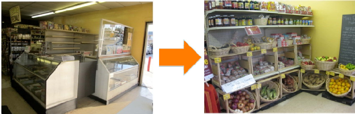
Basic produce installation from CRA/LA's Community Market Conversion Program Pilot. Estimated impact of store conversion: 13,500 households with expanded food access.
